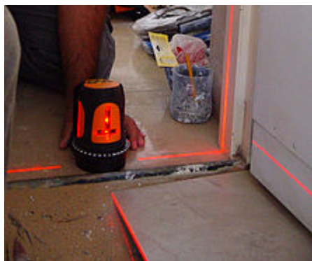
Levelling of ceramic tiles floor with a laser device
