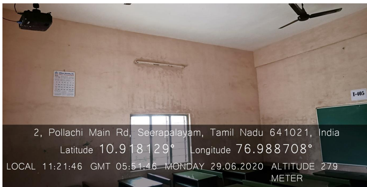
Figure E- 405- Class Room
