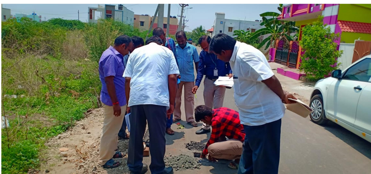
Checking the height of the pit
