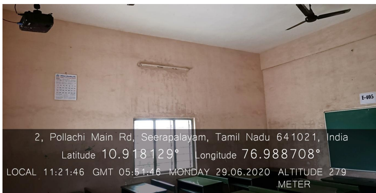
Figure E- 405- Class Room
